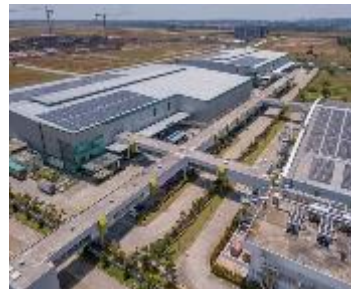
Solar Panel Support energy efficiency by installing solar panels in our new production facilities
